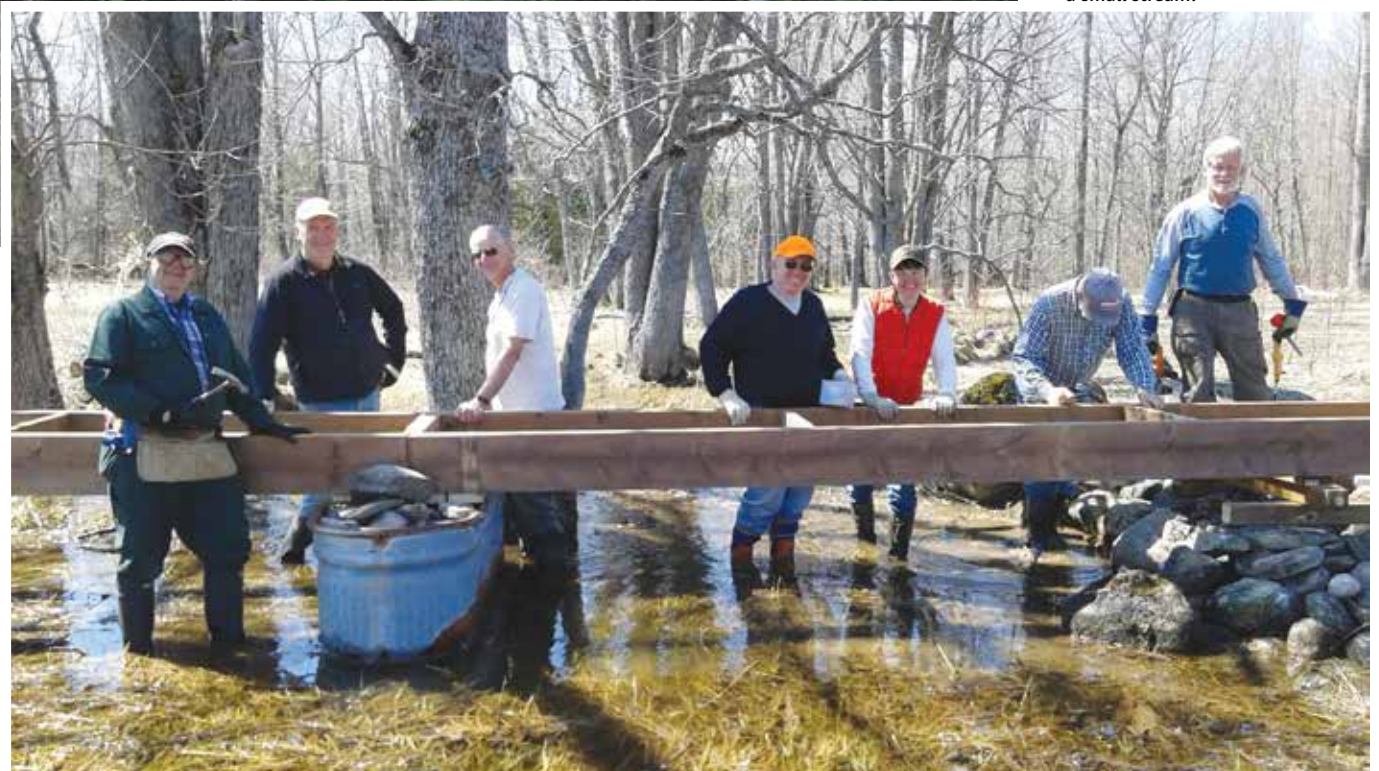
▼ Sydenham trail workers building a footbridge over a small stream.
