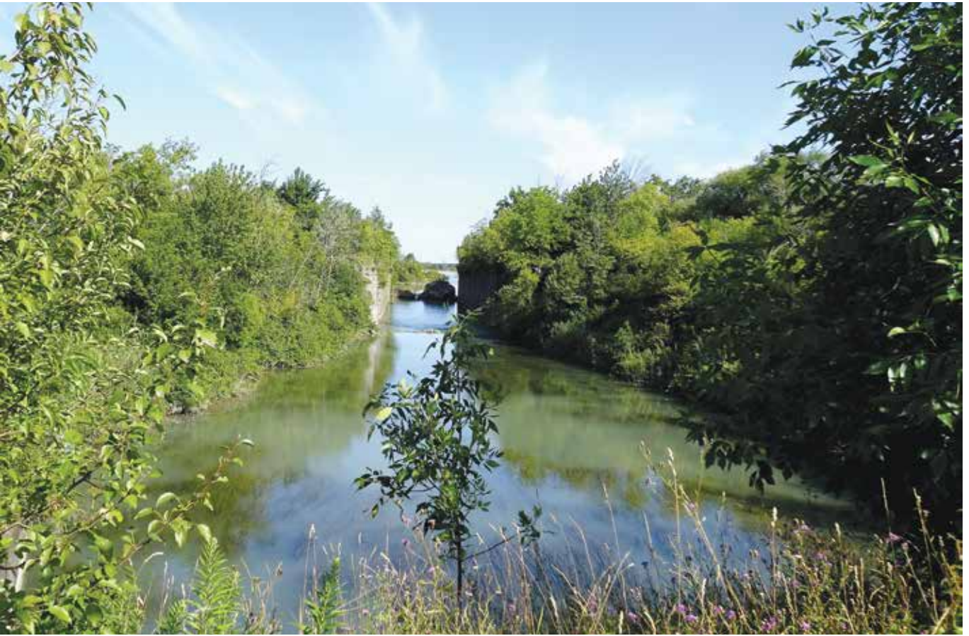
▲ This view looks north at Lock 12 of Canal #3. This is the last accessible lock before this canal turns west to cut diagonally across St. Catharines. The next accessible lock is 4 on the far side of the city. Open water in the background is a reservoir for the current canal, #4.
