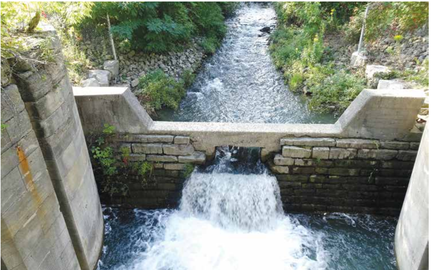
▲ Lock 8 of Canal #2 is well preserved and shows the contouring of the stones to accommodate wooden gates. This view looks south from a narrow footbridge.
