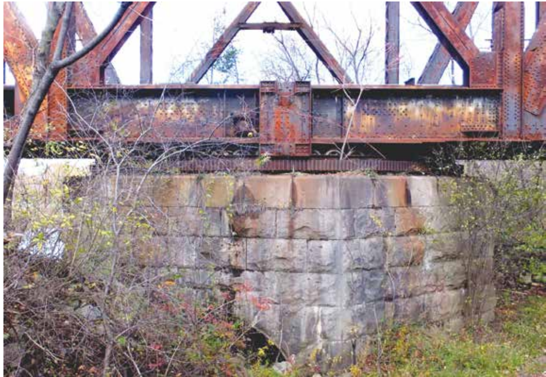
▲ Built in 1887, this double-track steel bridge is still used today by CN Rail. The enormous steel gear used to drive the bridge when it rotated to allow ships to pass.
