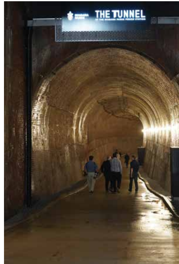
▲ The Tunnel is a pathway 180 feet below ground, inside the former waterway to the Niagara River. Visitors walk the 2,200-foot channel to reach the viewing platform.
