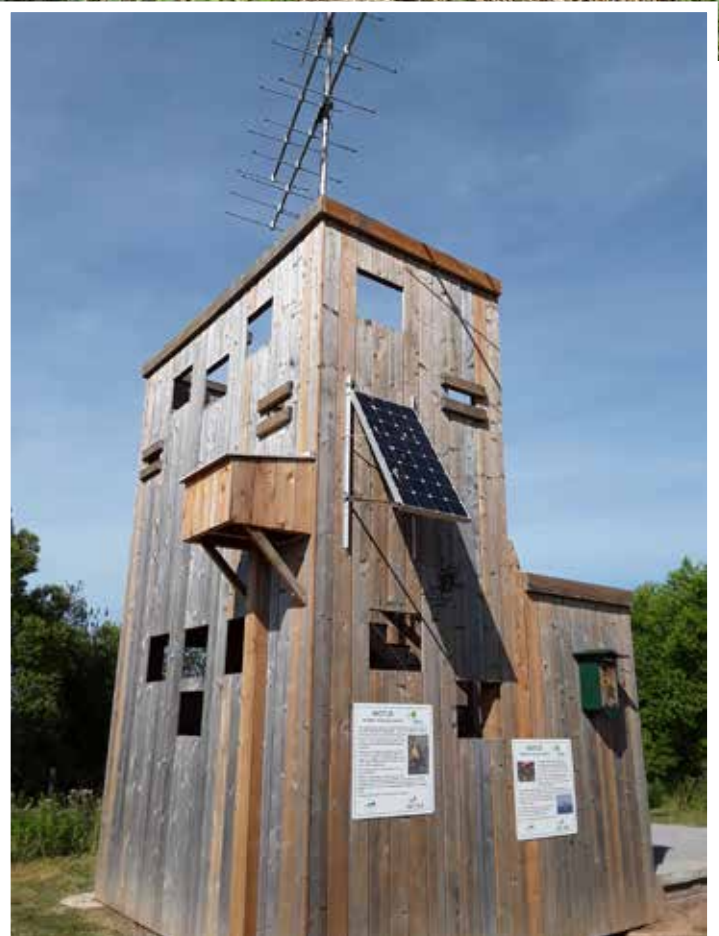
► The completed two-storey wildlife observation structure has a radio tracking tower that uses the specialized Motus program to collect data on migrating creatures.
