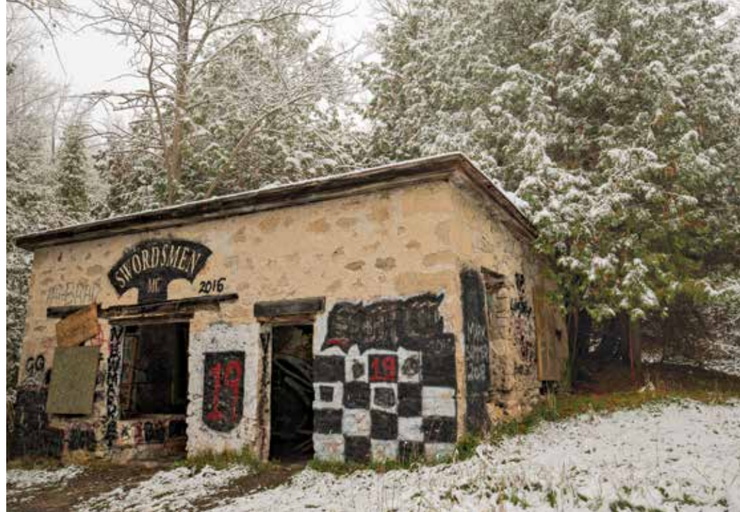
▼ Walkers pass this stone building above the falls, which was built in 1895 by William Hogg. It was the power house containing two turbines that generated enough power to provide electricity to the town of Eugenia and nearby Flesherton. It sits in poor condition.
