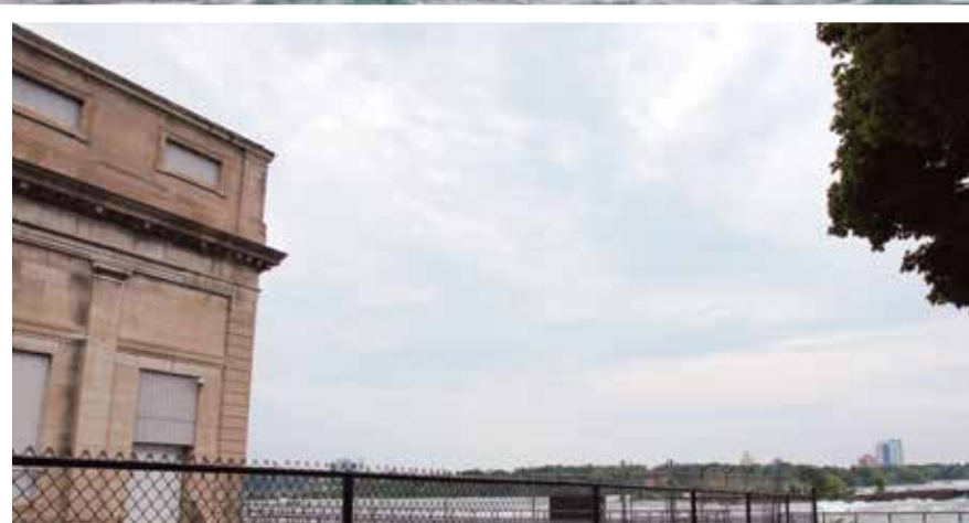
◀ A corner of the power house. In 1918, lines were sent from the roof over to the iron scow, lower right.
