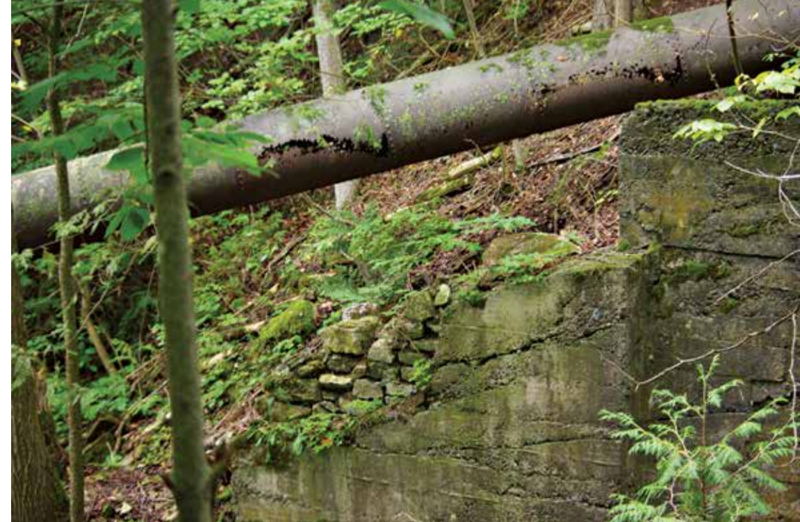
▲ William Airth Mill at Horning Mills was leased by John A. Plewes of Kimberley in 1867. The penstock can still be seen on the far side of the Pine River, about 150 m downstream from the mill pond dam.
