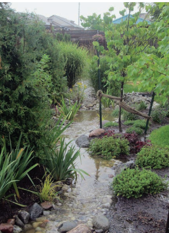
◀ Rain gardens hold and infiltrate water in a beautiful way, helping to preserve our creeks. It's important that they drain in 24 to 48 hours.
