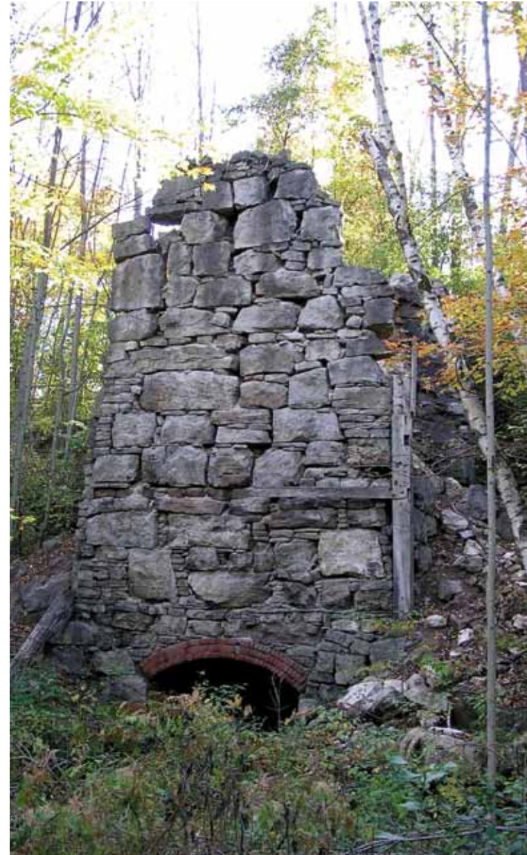
▲ Looking like a temple found in a tropical jungle, this is the ruin of the Draw Kiln before research and restoration.
