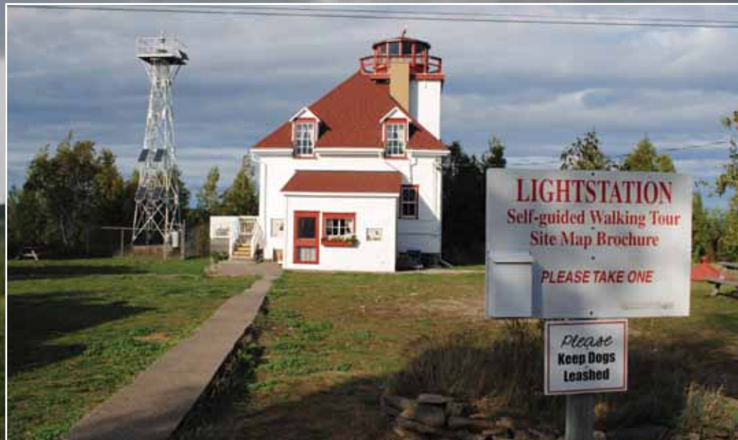
▲ Cabot Head Lightstation, old and new. Today's automated, solar-powered navigational beacon stands atop a steel tower adjacent to the original, wooden lighthouse structure built in 1895.
