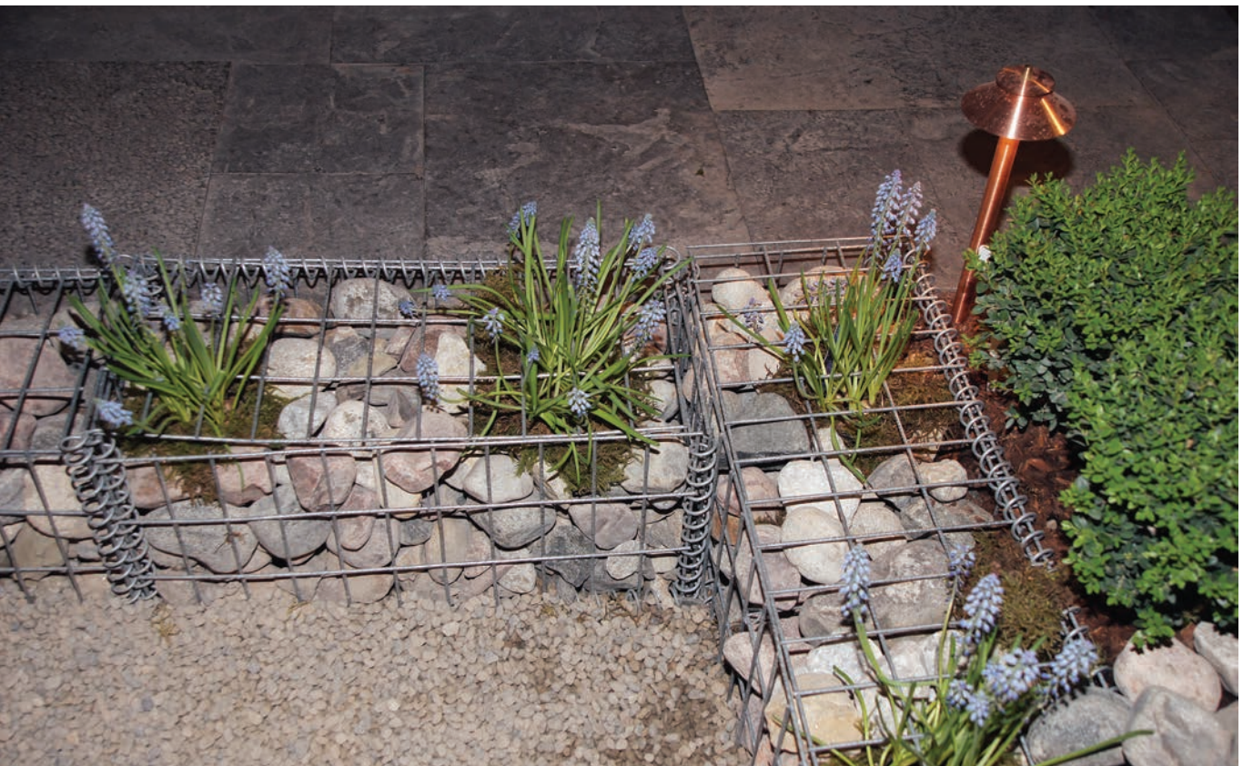
▲ Gabion baskets filled with rocks formed a retaining wall. Grape hyacinths were planted in soil pockets among the rocks.
